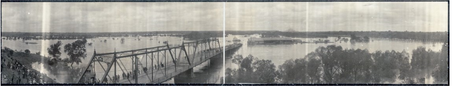
[ photo of 1908 flood ]
